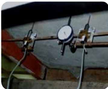
Fig. 6 – Units of (LVDT) under the slab
