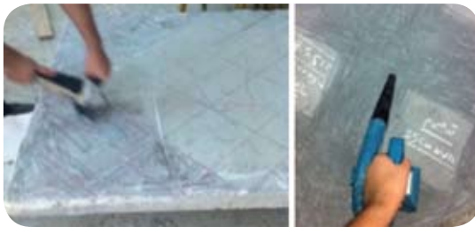
Fig. 1 – Scraping and removing dust and fine materials with compressed air
