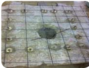
Fig. 4 – 8 steel bars in each direction fixing 16 steel screws
